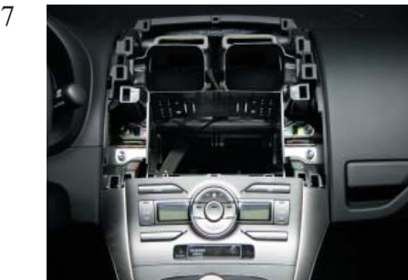
Place the metal bracket into the dashboard between the metal OEM brackets.
